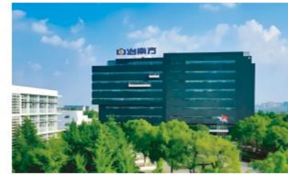
MCC South (Wuhan) Automation Co., Ltd.
