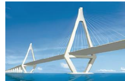
Guangdong-Hong Kong Cross-Sea Bridge
