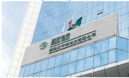
Liaoning Provincial Power Company
