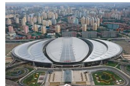
Beijing South Railway Station
