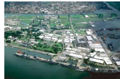
Subic Bay Solar Power Plant Philippines
